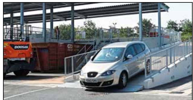
Job done... residents enter and leave the deck by ramp sections that are part of the Modulo-Beton “kit”.
